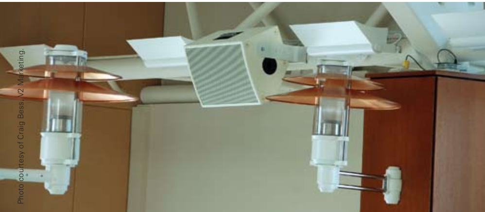
Photo (left): Westover features a full complement of Electro-Voice loudspeakers controlled by EV's new NetMax digital audio system controller.
